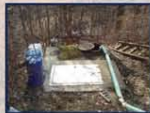
Pre-Upgrade Chlorine Contact Tank
