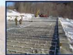
RSF During Construction
